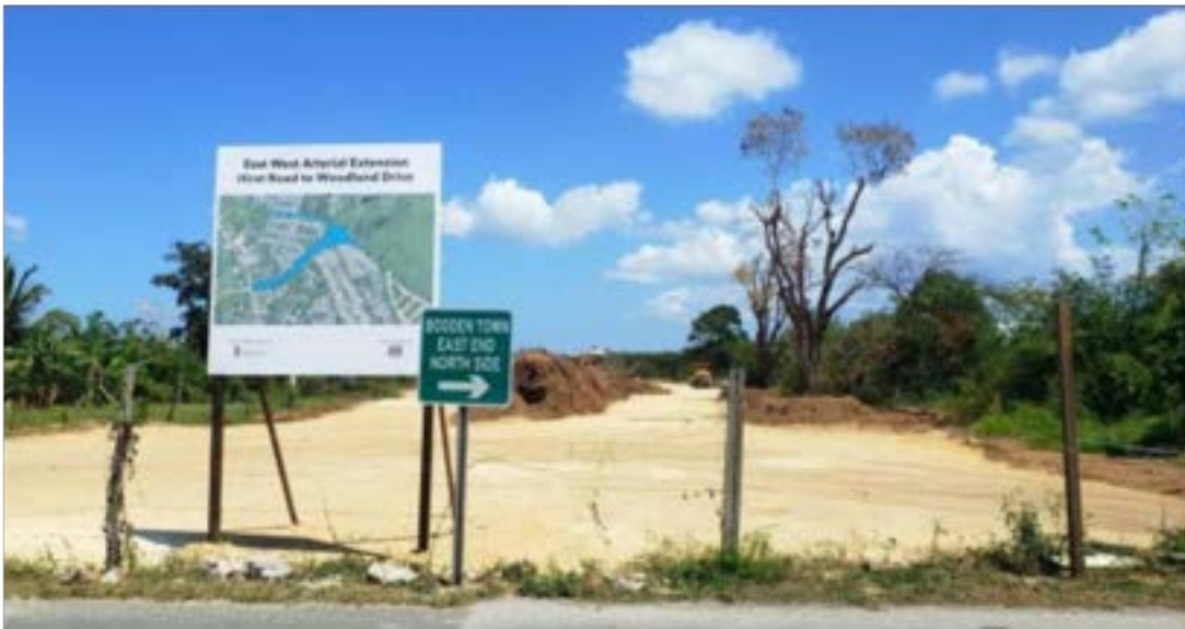
The East West Arterial Project. Photo Credit: National Roads Authority.
