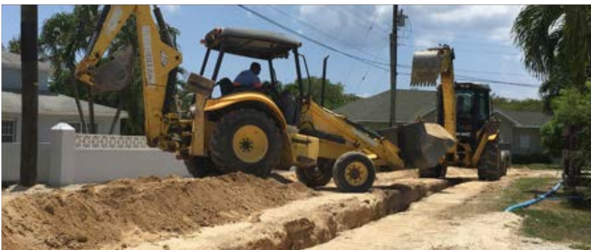
Water Authority crews conducting roadworks in the Bodden Town.
