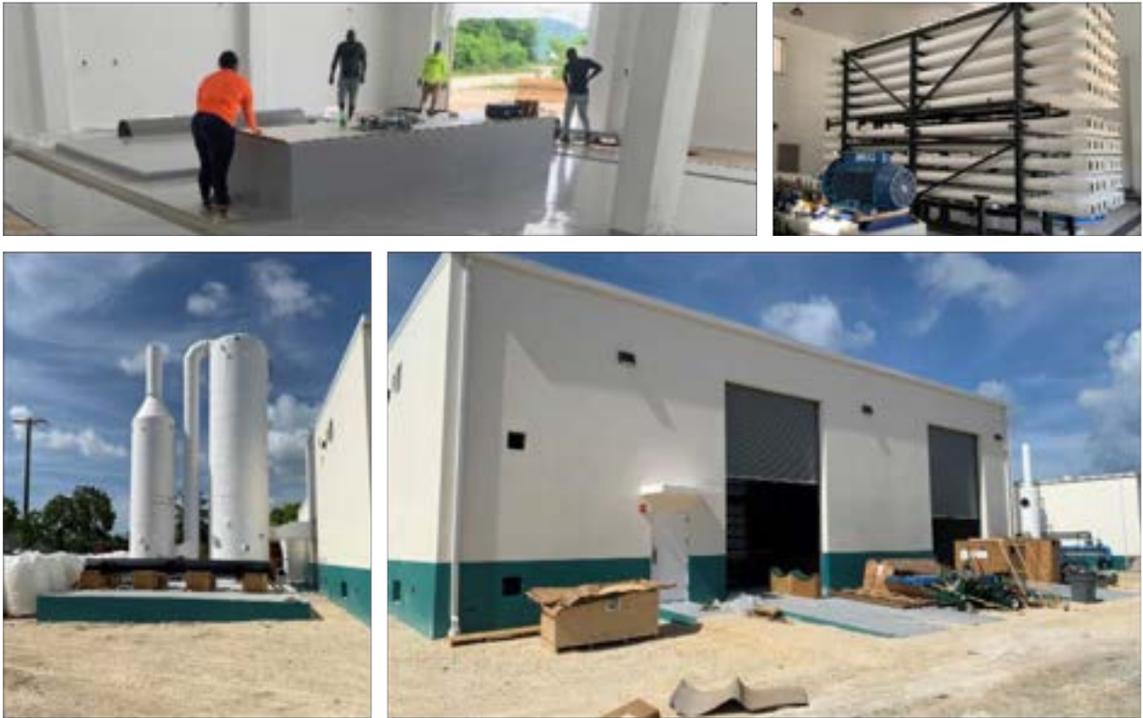
Construction process of the new RO Plant.
