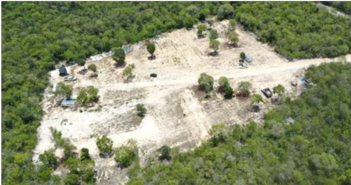
The site of the future Bluff Water Works in Cayman Brac.
