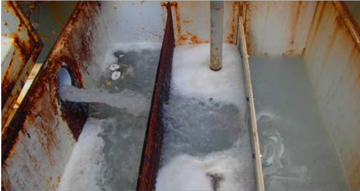
Testing at a substandard treatment plant.
