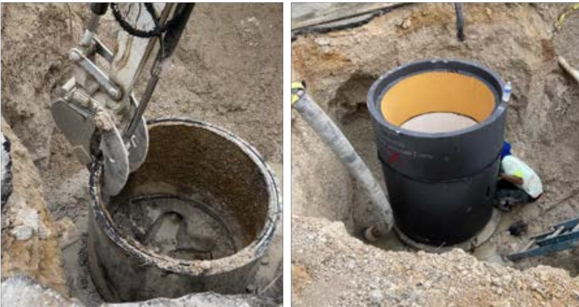
A before and after of a manhole that was rehabilitated in 2023.
